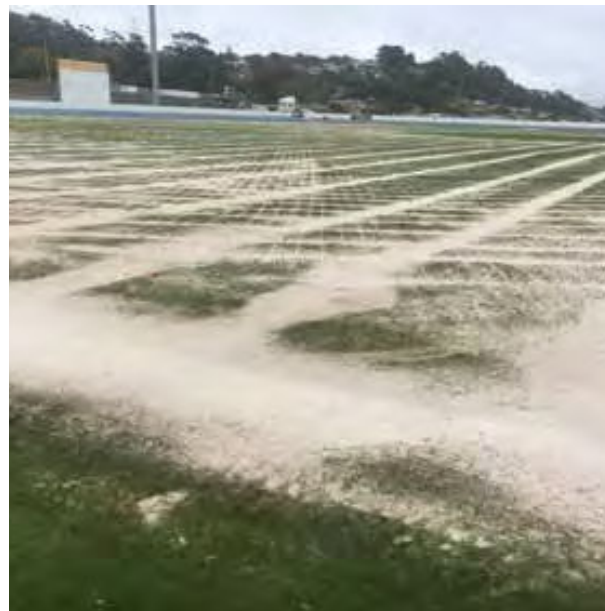
Installing sand slit drains into existing sportsfield
