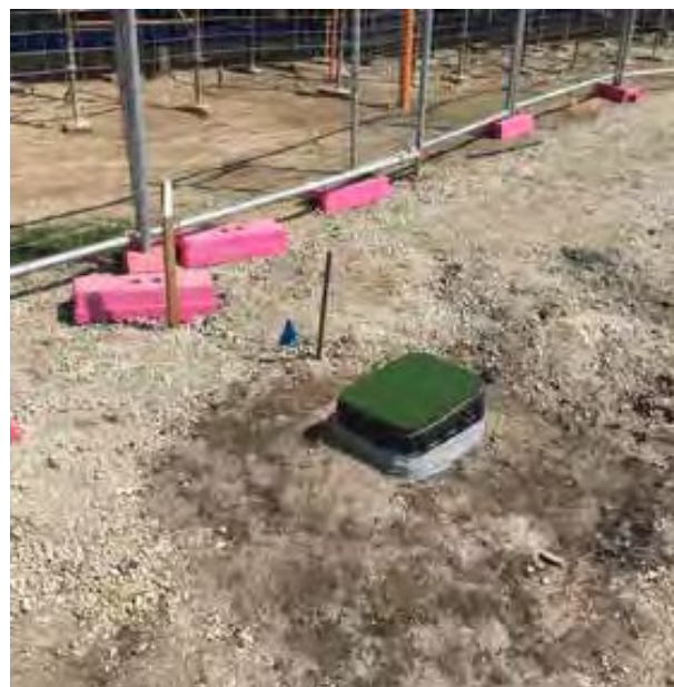
Installed solenoid box
