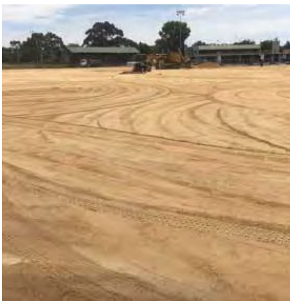
Installation of sand root zone layer
