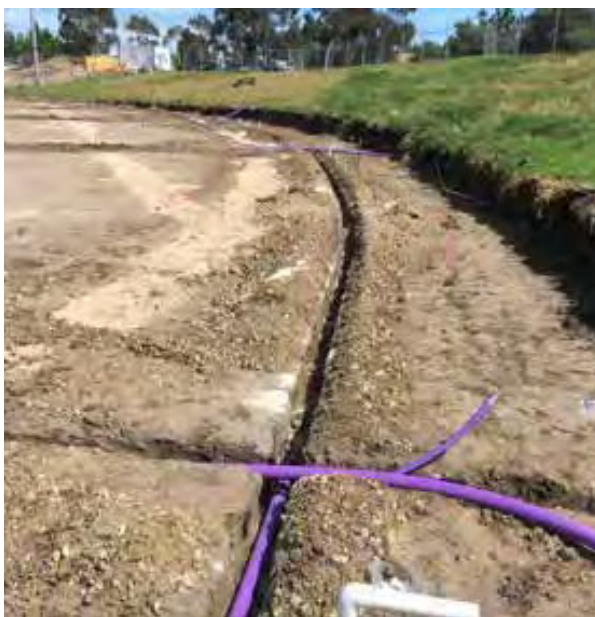
Installation of irrigation pipework
