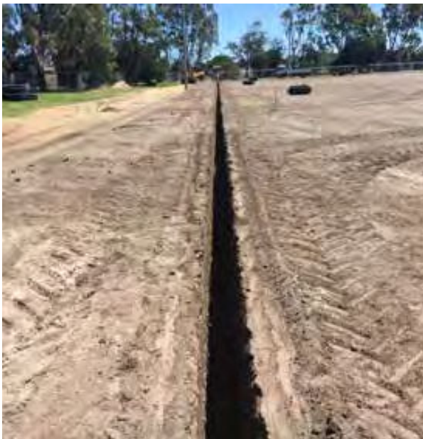
Trench dug prior to installing drain
