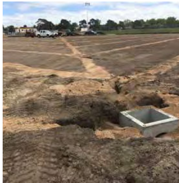
Subsurface drainage being installed in oval
