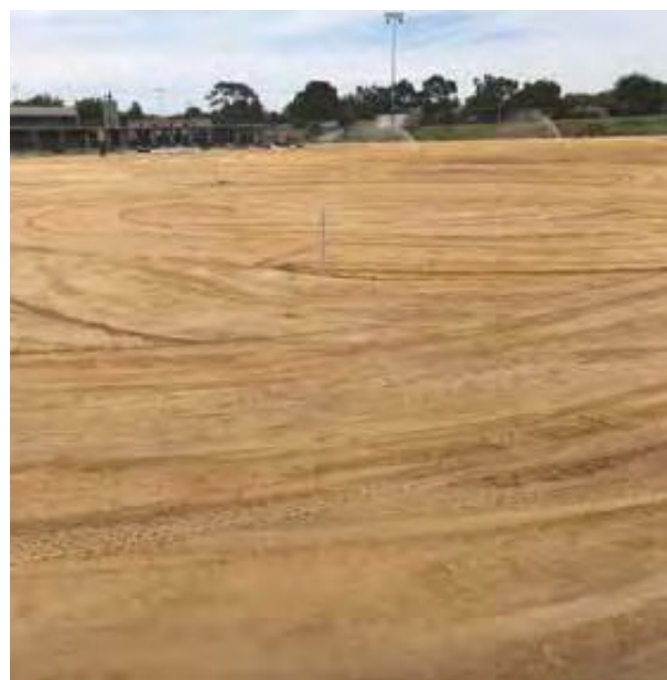
Installation of sand root zone layer
