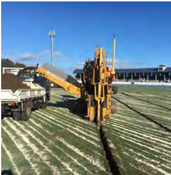
Installing sand slit drains into existing sportsfield
