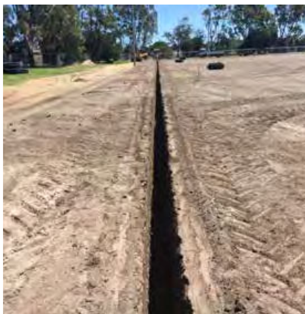
Trench dug prior to installing drain
