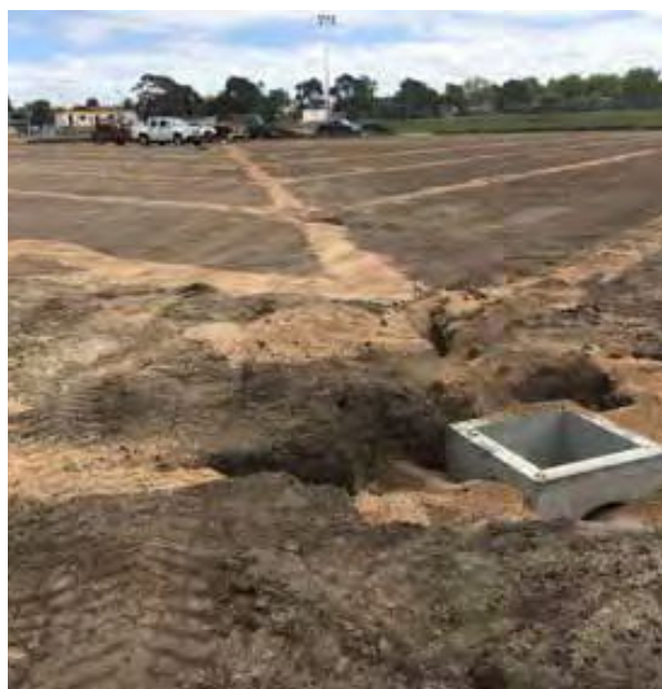
Subsurface drainage being installed in oval
